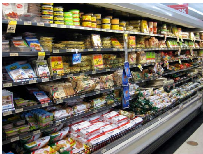
Figure 1.5: An example of open vertical display cabinets
