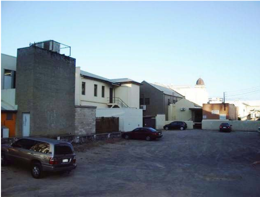
Denham St frontage.
