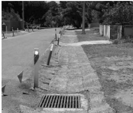
Figure 7.3.6 Retrofit of Street with a Swale, City of Onkaparinga.
